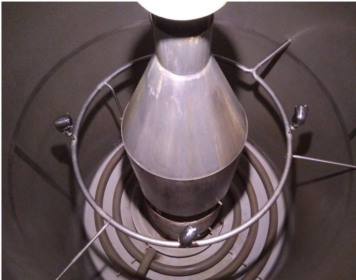
*Figure 2: The four Bio 10s inside the Ringwood 'copper'*
